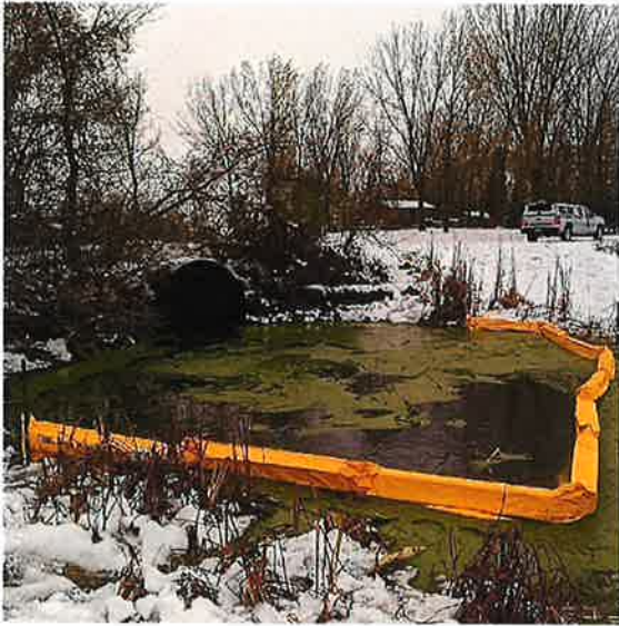
Floatation silt fence installation.
