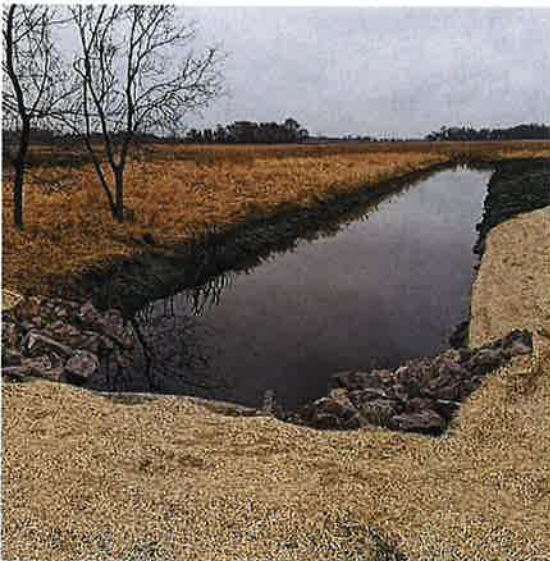
Typical seeding and blanketing procedure.
