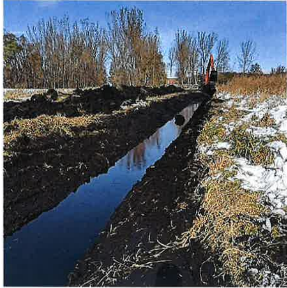
Typical ditch cleaning.
