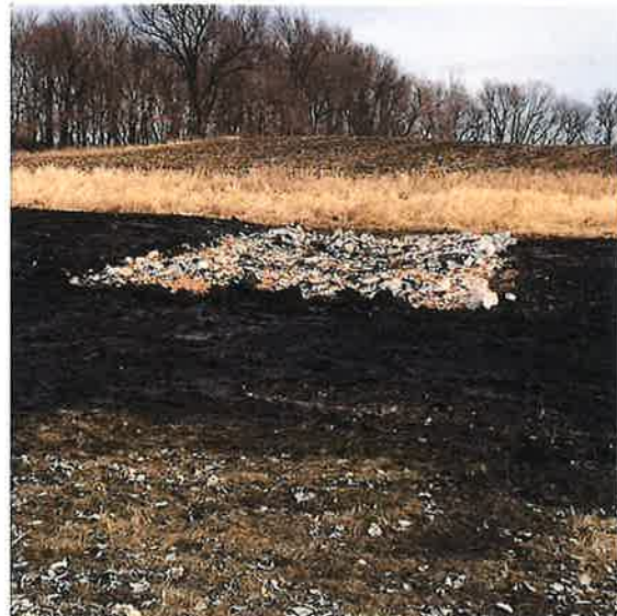
Typical spillway overflow rip rap area.
