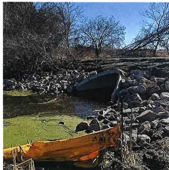
Finished road crossing at 0+00 with rip rap North side.
