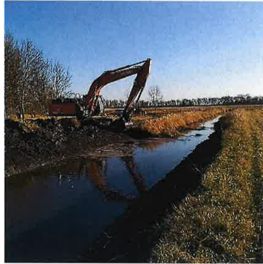
Typical open ditch cleaning.
