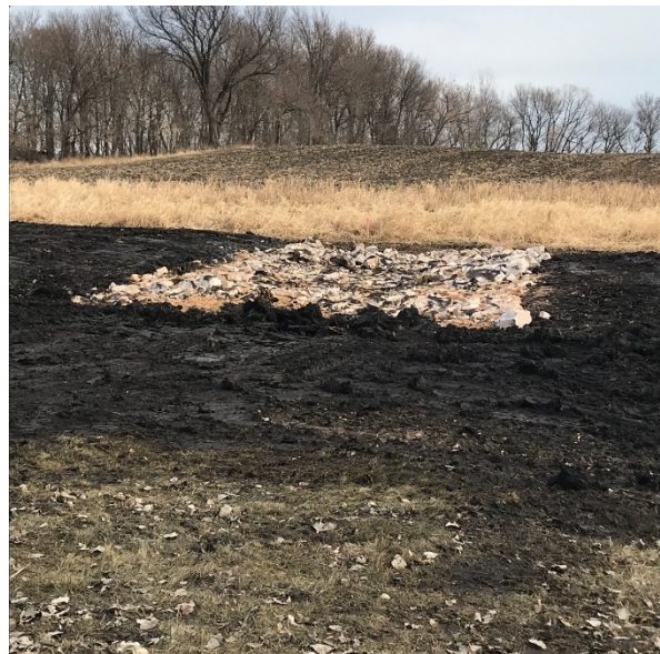
Typical spillway overflow rip rap area.
