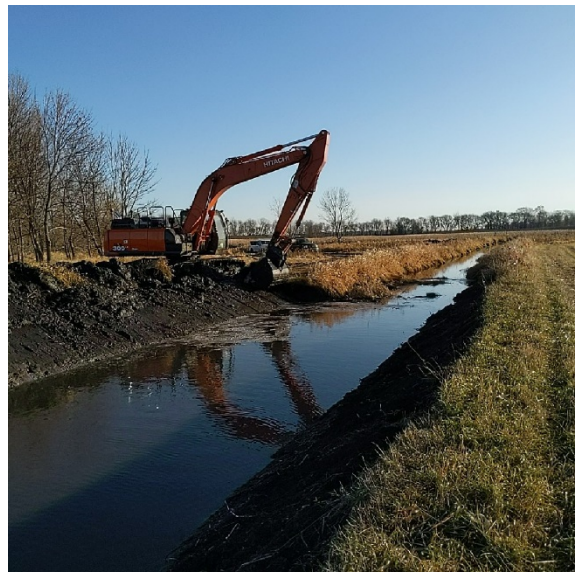
Typical open ditch cleaning.
