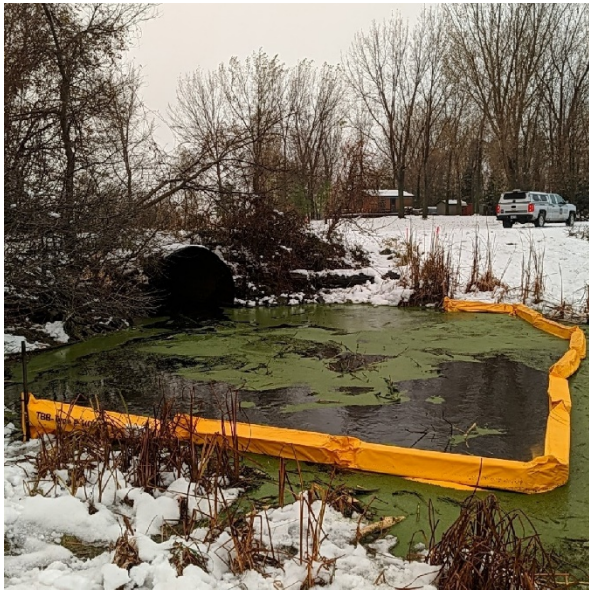
Floatation silt fence installation.
