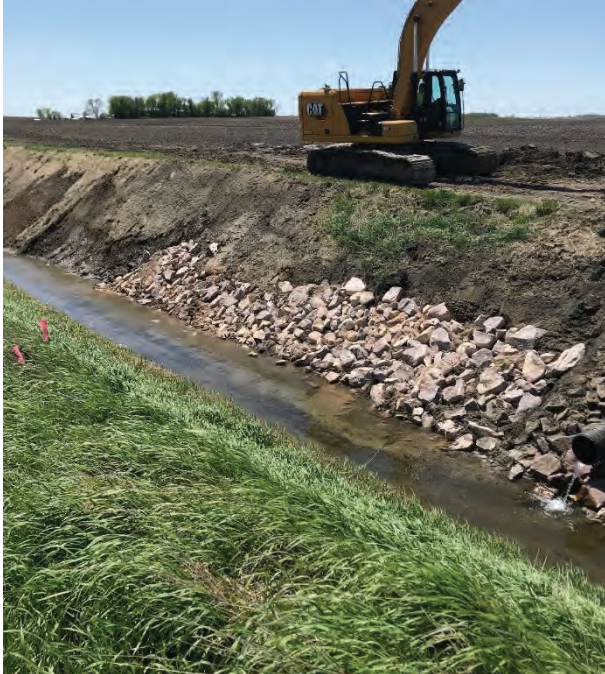
TYPICAL BANK ARMORING WITH CLASS III RIP RAP.
