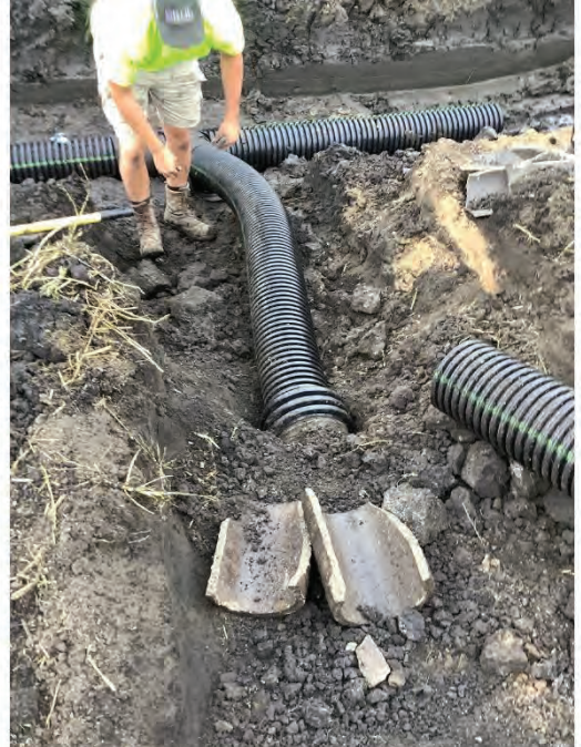
TYPICAL PRIVATE TILE CONNECTION INTO NEW 10" SUB MAIN.
