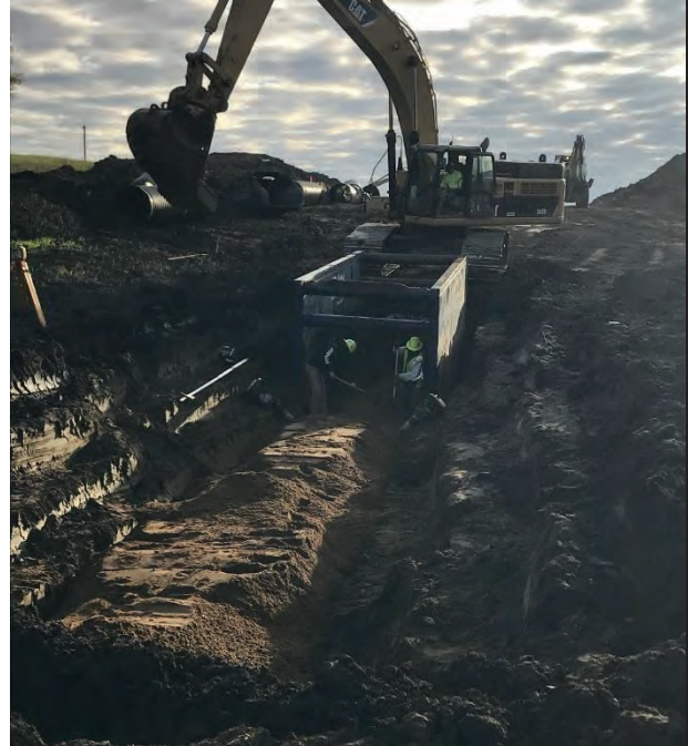
TYPICAL PRIVATE TILE CONNECTION INTO NEW 10" SUB MAIN.
